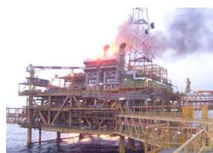
Figure 6 - Fire ignition due to DGS failure
